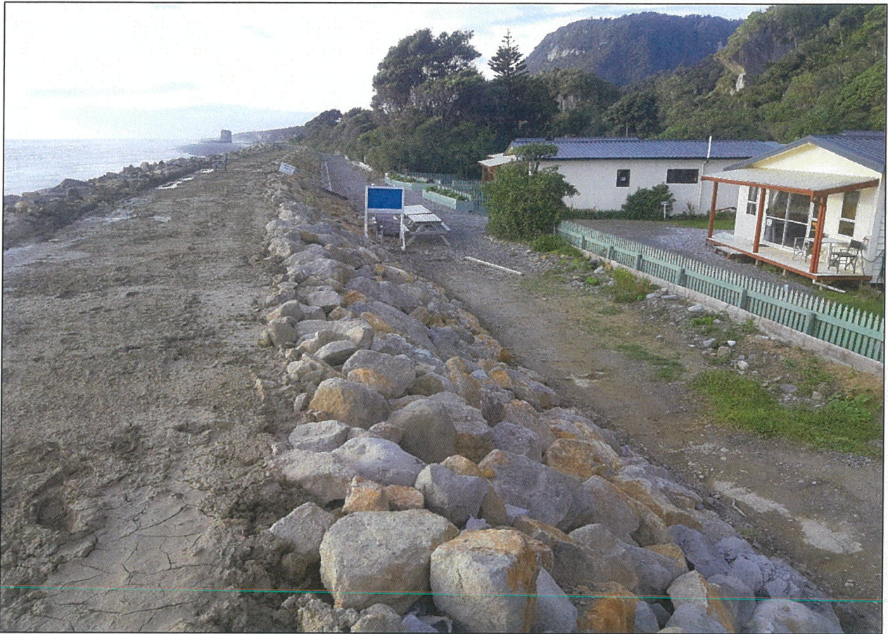
Rubble riprap placed on the lee-side of the wall.
