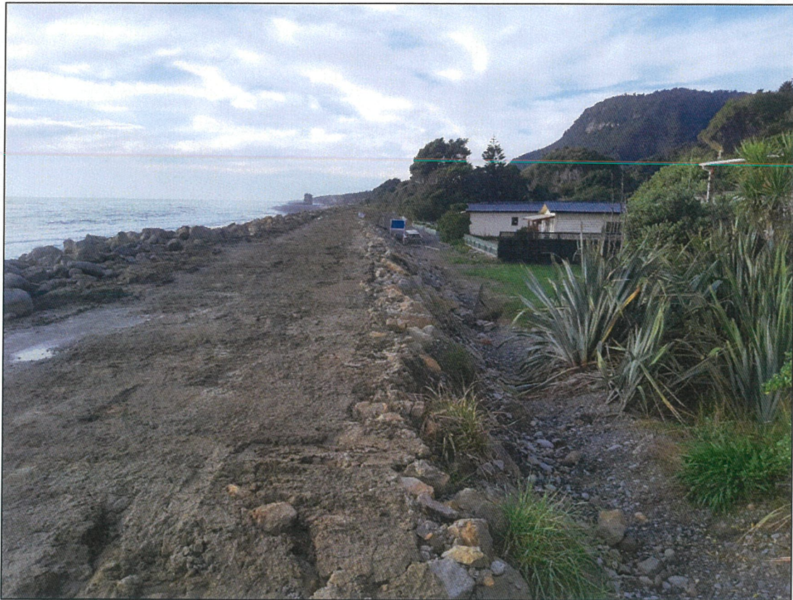
Looking north from the boundary of the seawalls.
