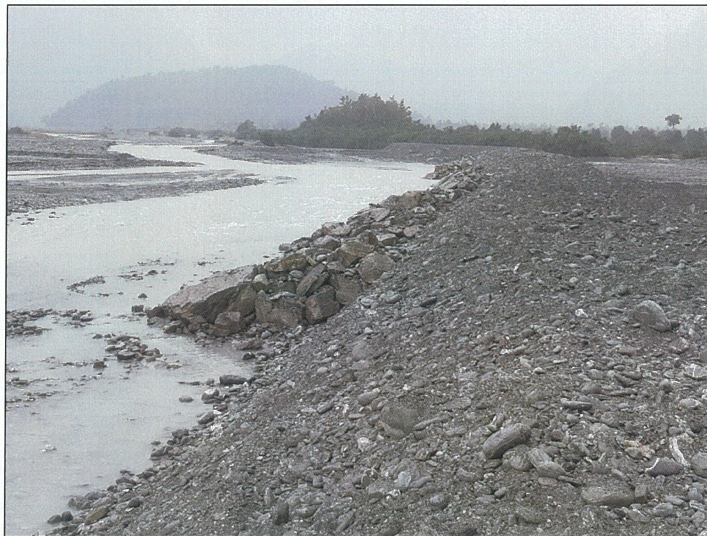
Temporary Diversion Wall
